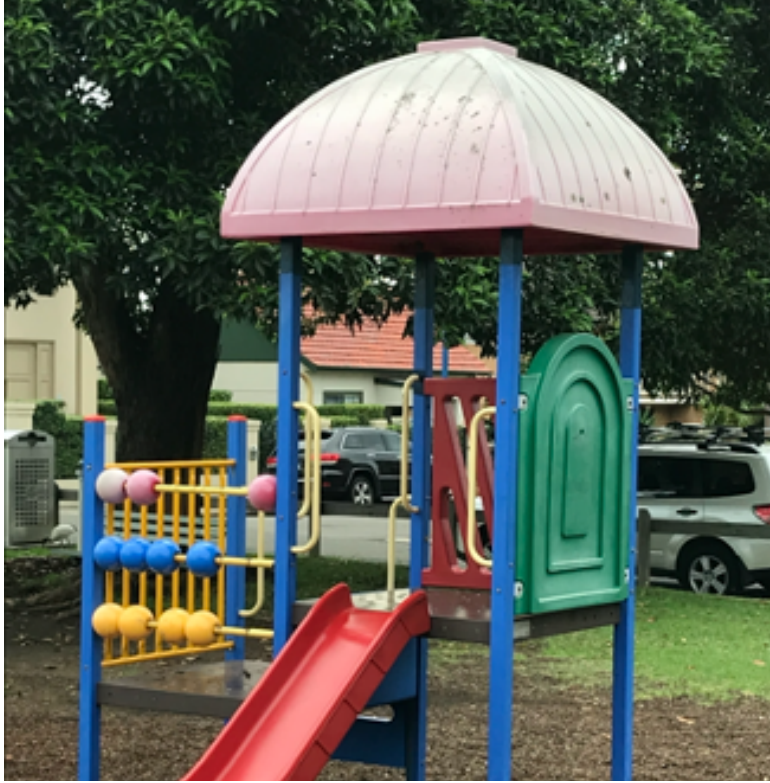
Figure 24: Appropriate shade would have protected this play equipment from the damaging effects of UV and a degraded visual appearance, prolonging its useful life. Photo: from the project image bank, collected by the research team during site visits.
